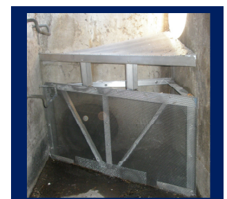
“Grate Trash Catcher” CPS: Effective in catch basins as small as 18” x 18” x 18”
