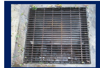
“Grate Trash Catcher” CPS: Effective in catch basins as small as 18” x 18” x 18”
