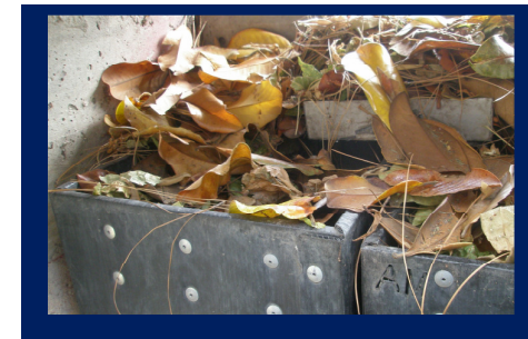
Competitor's boxes fill with debris impacting filter effectiveness. Choose Waterway Filter boxes with slanted, screened opening to keep out trash.
