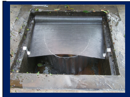
“Wavy” Corrugated CPS: Increased effectiveness in a smaller footprint
